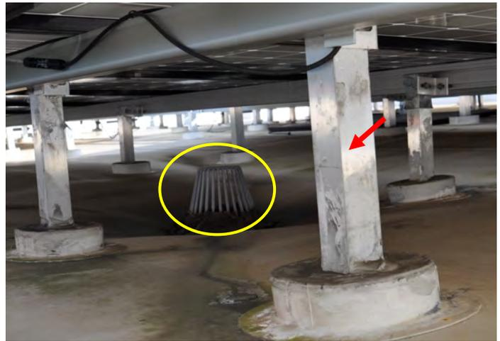
*Figure 10 PV panels extended over this roof drain (yellow oval), thereby making it difficult to check for dogging and removal of debris. The red arrow indicates a rail support post.*
