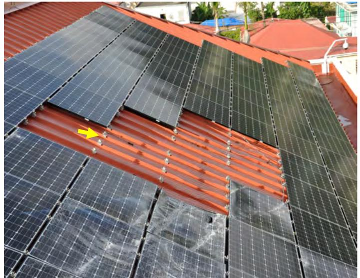
*Figure 12. These PV panels were attached directly to the standing seam ribs with panel clamps that were attached to external seam clamps (yellow arrow). Note that several panels in the foreground were damaged by wind-borne debris (reportedly a collapsed antenna).*
