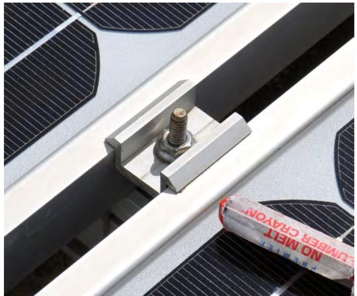
*Figure 13. View of a PV panel clip after the 2017 hurricanes. Although there was no apparent loosening of the nut, the bolt could be wobbled with finger pressure. A loose nut such as this is susceptible to further loosening and loss of the clamp's ability to keep the panels in place.*
